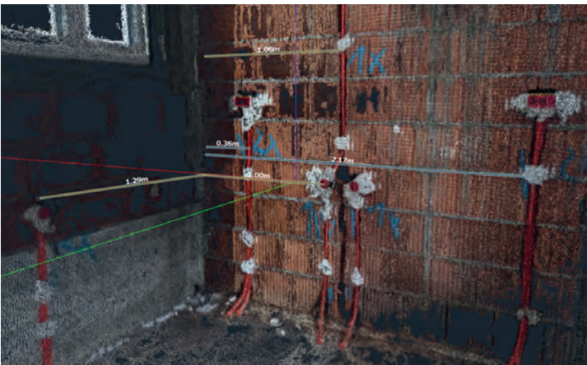
▲ Figure 6: Indoor survey showing electrical conduits.
